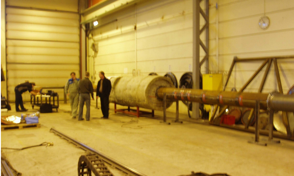
fig 2. Photo for duct before and after silencer
